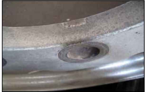
Galvanic corrosion in wheel nut area and inside center bore
